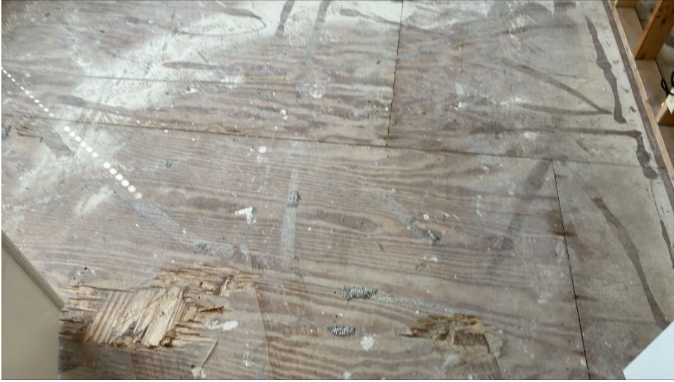
Guest bedroom, subfloor
