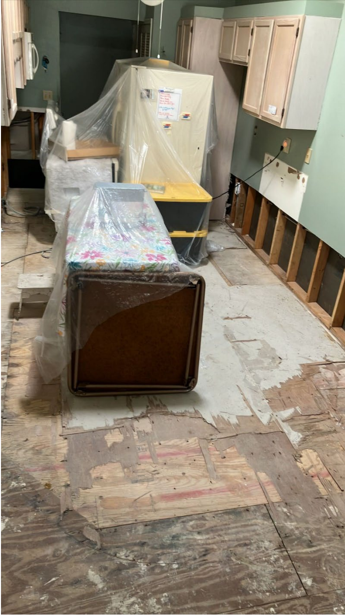
Sub flooring in kitchen
