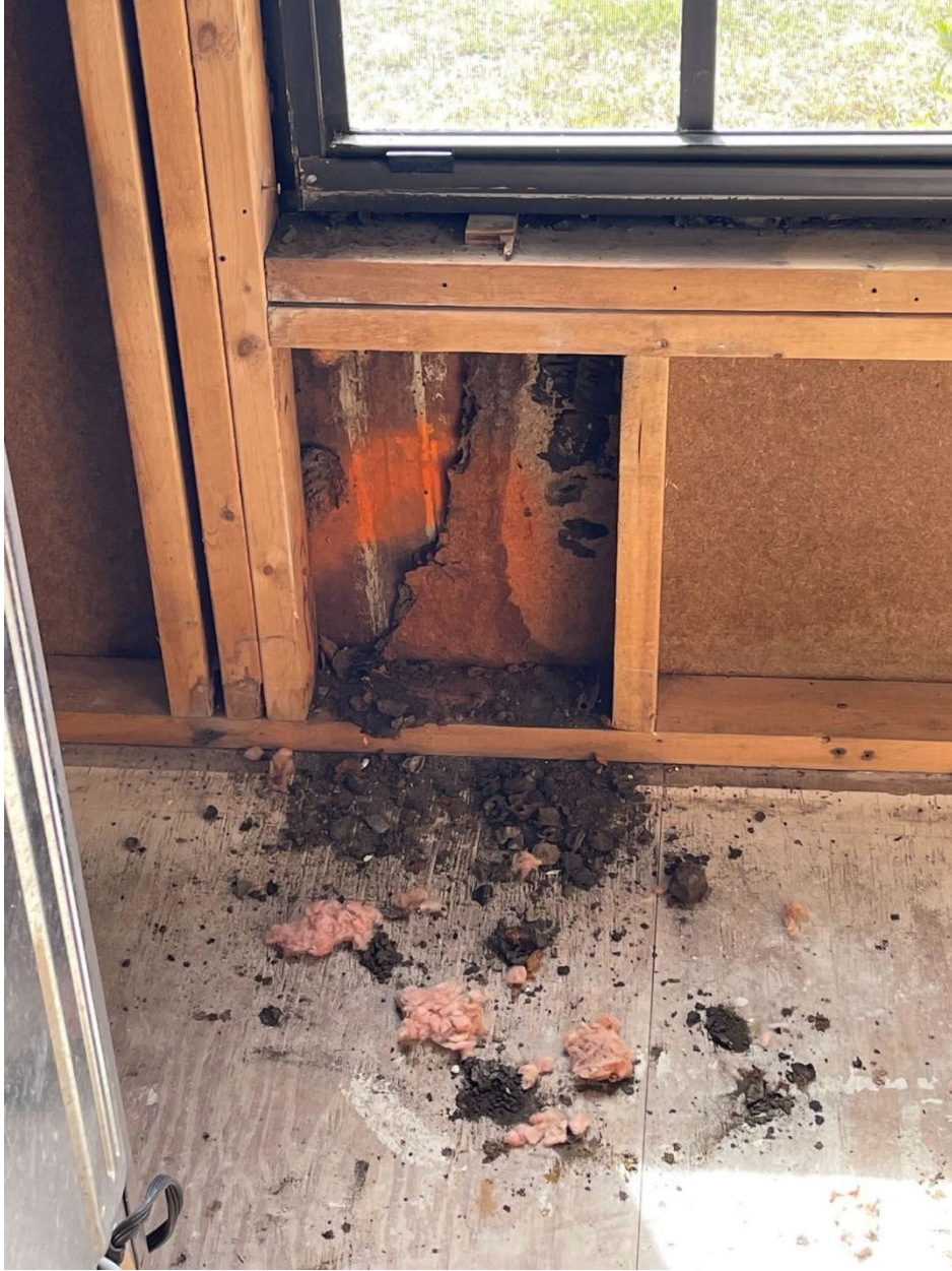
Under living room window, wood sheathing
