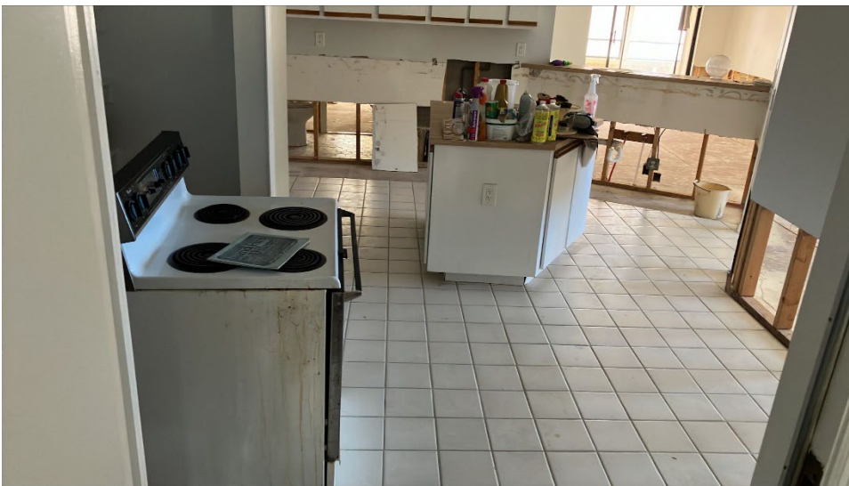
Kitchen sub floor removal
