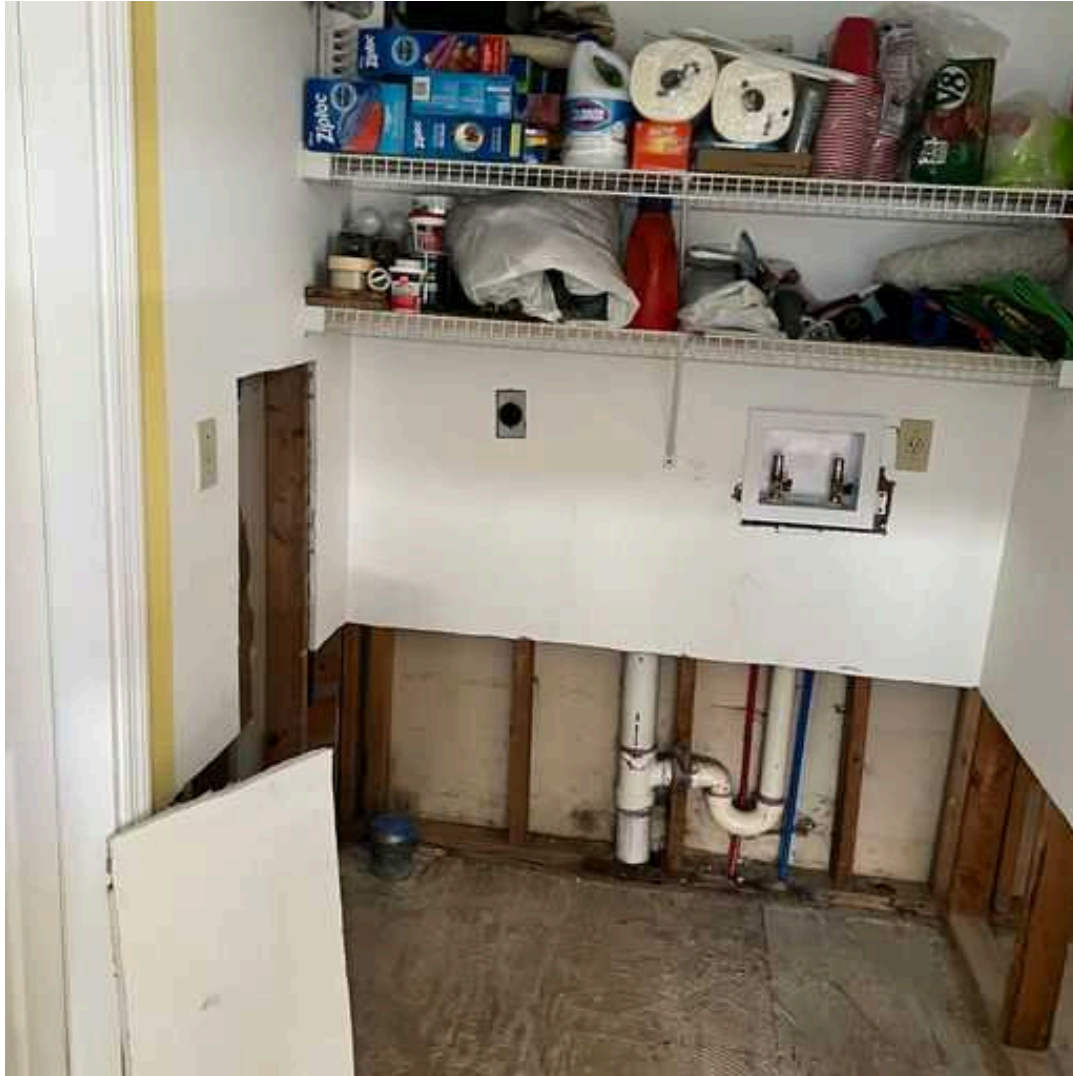
5 Main Level/Laundry Room - 3- Laundry room
