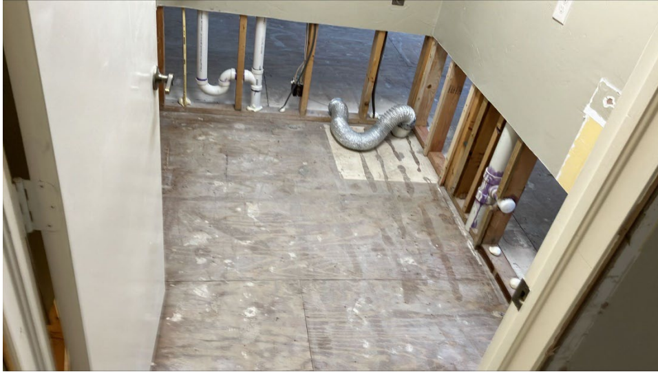
Laundry room subfloor
