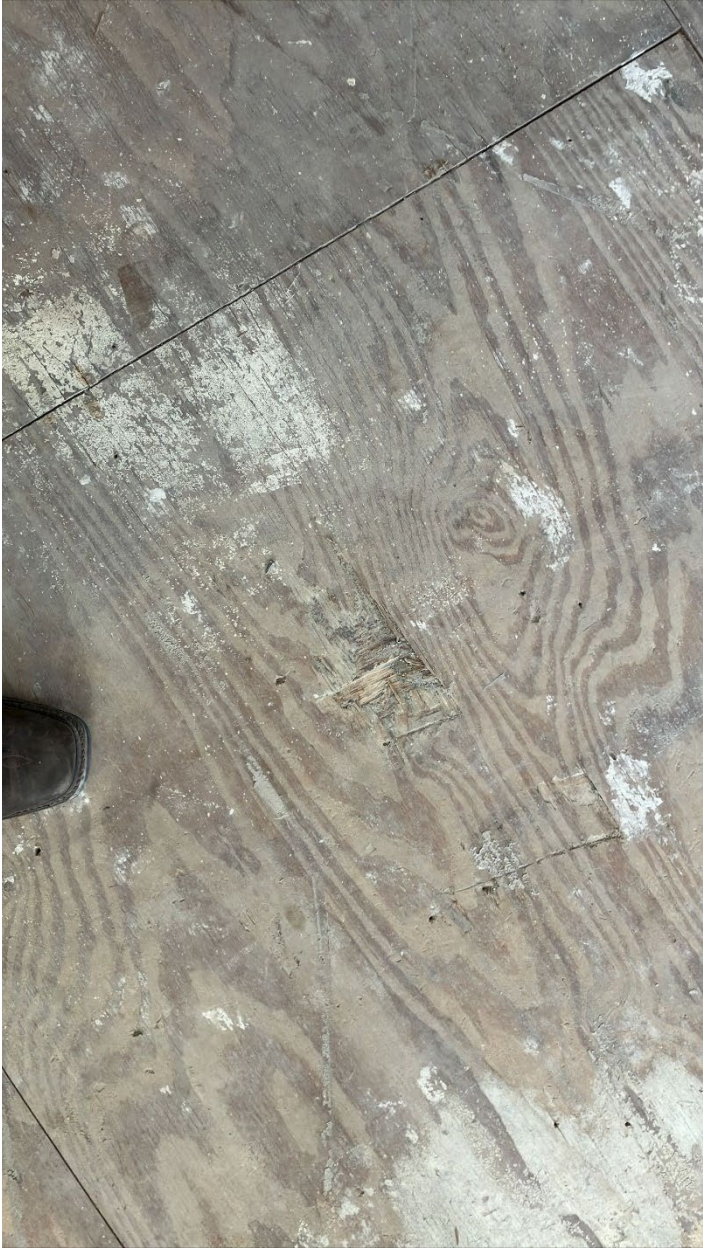
Chipped up sub-floor
