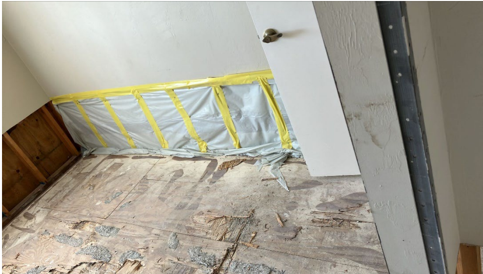
Subfloors guest bedroom two
