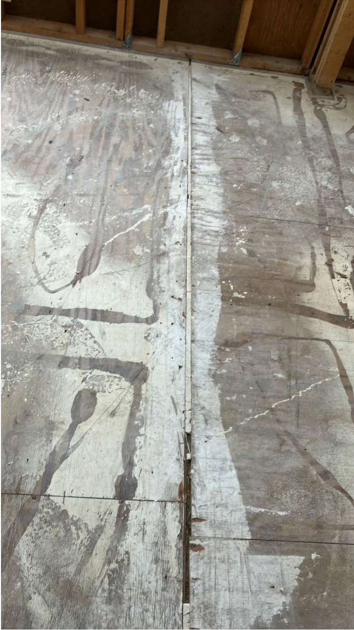
Guest bedroom one subfloor
