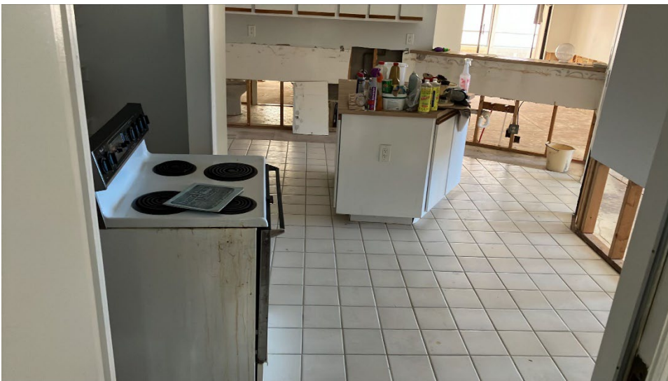
Kitchen sub floor removal
